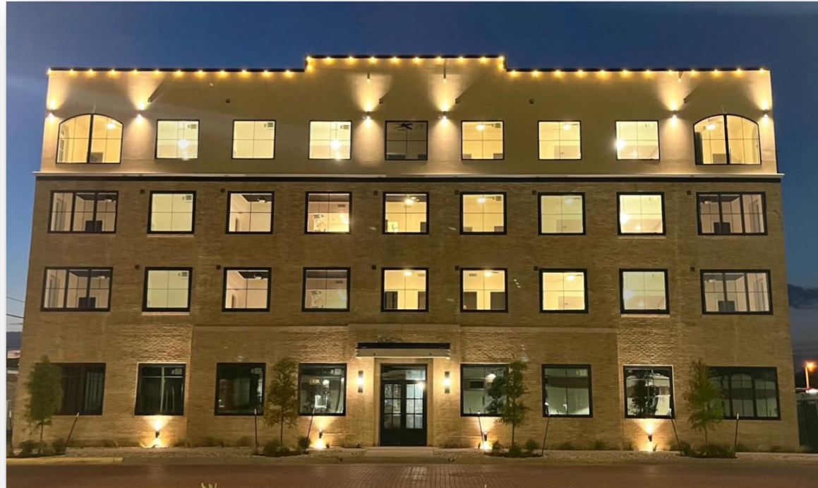
The Wyatt. Stephenville, TX Mixed-use Historic Redevelopment 2024
