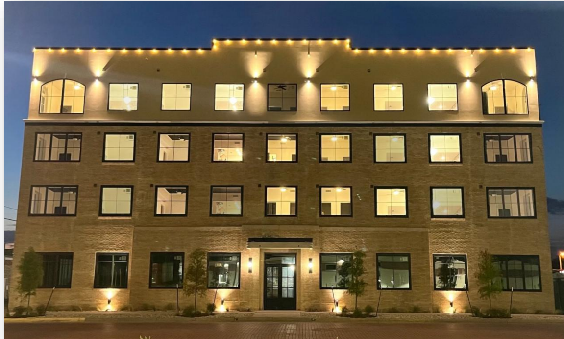
The Wyatt. Stephenville, TX Mixed-use Historic Redevelopment 2024
